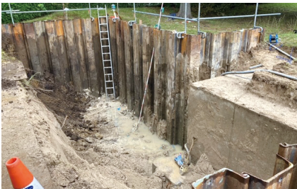
Excavation and removal of contaminated soil (former Advanced Materials Research Laboratory of Toyo Ink SC Holdings Co., Ltd.)
